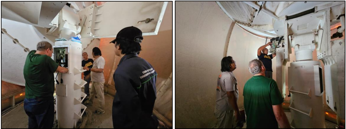
Gambar 36. Preventive Maintenance Radar Cuaca
